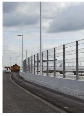
on the barrier actually breaks down the NOx and VOC into harmless by-products. It also reduces noise.
